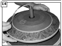
Thread wires and safety cable through upper body and install over downrod to fan body. Next thread wires and safety cable through canopy and place over downrod.
